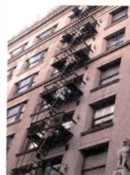
6 a fire escape
