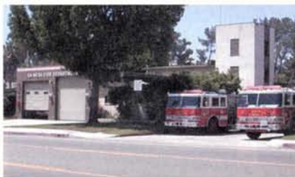
3 a fire station
